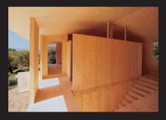
They are produced in a maximum length of 16.50 m, a maximum width of 2.95 m and a maximum panel thickness of 0.50 m subject to constant internal and external supervision.
