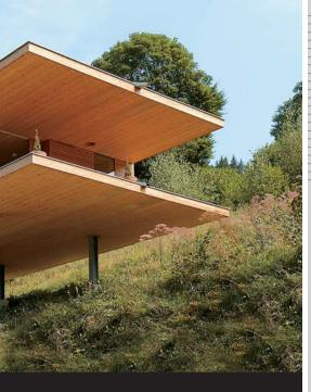
The large formats of the KLH solid timber panels, the cross lamination, the structural capacity and the possibility of combining it with steel, glass etc offers ultimate design freedom - from detached houses, multi-storey residential blocks and public and commercial buildings to arched roofs and bridge constructions.
